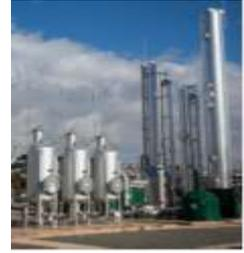
Energy blending eliminates the requirement for propane addition. However, the autonomous detection of blended gas outside legal tolerances results in liquid propane injection from a 12 tonne reserve stored above ground.
