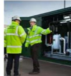
Pressurisation of biomethane occurs on site with the use of a single phase Wartsila oil free compressor. A compression of up to 20 bar is achieved prior to delivery into the lower transmission system.
