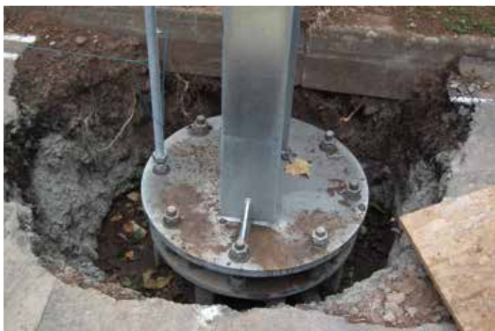
Steel pins for installing with concrete piles Photo courtesy of Evoenergy
