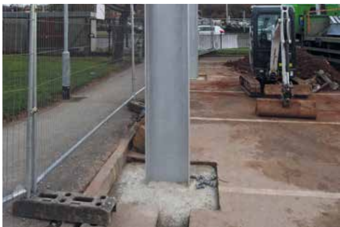
A concrete footing, photo courtesy of EvoEnergy
