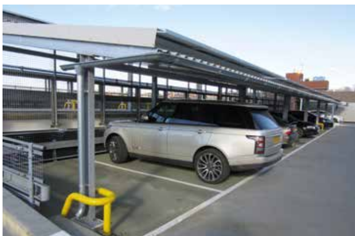
Guttering attached to a downward column Photo courtesy of SunGift Energy
