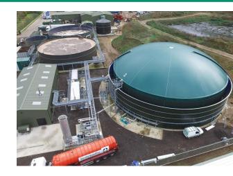
What are the estimated carbon savings?: Using 400m3/day of liquid process residues & 20 tonnes/day of solid bio-wastes, the plant is reducing the site's emissions by circa 20%.
