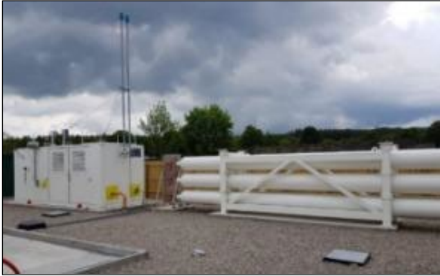
PRMS (250 – 2barg) and Bio-CNG Storage
