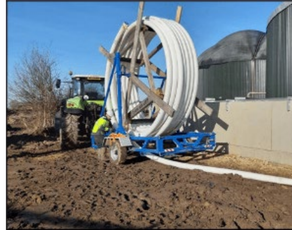
75 bar Soluforce Pipeline
