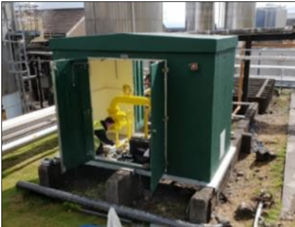
Final 2 bar to 200 mbar Regulator
