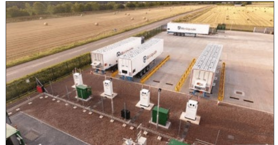
Bio-CNG trailers being Filled
