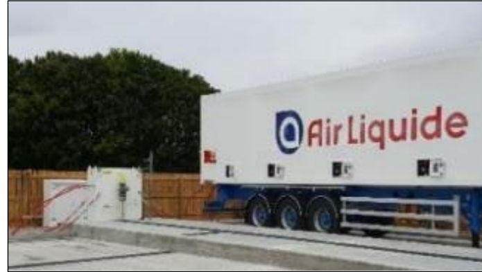
Offloading Cabinet and Bio-CNG Trailer
