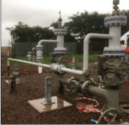
Connection at 85 Bar Block Valve
