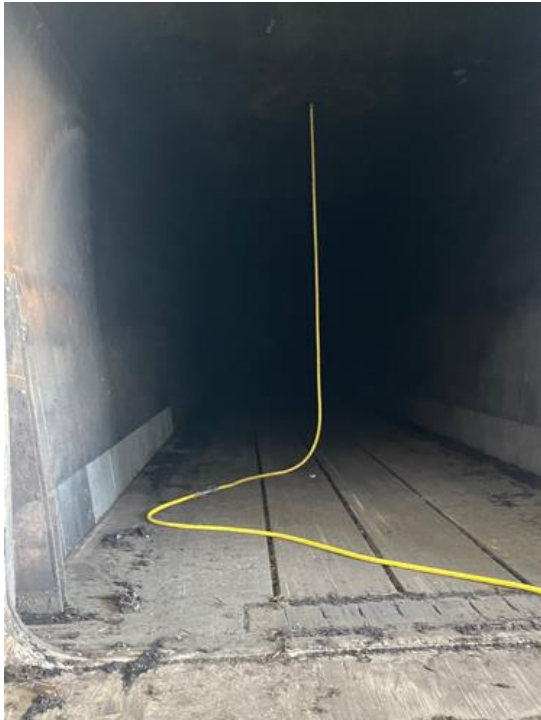
Photo 5 - Empty digestion tunnel
